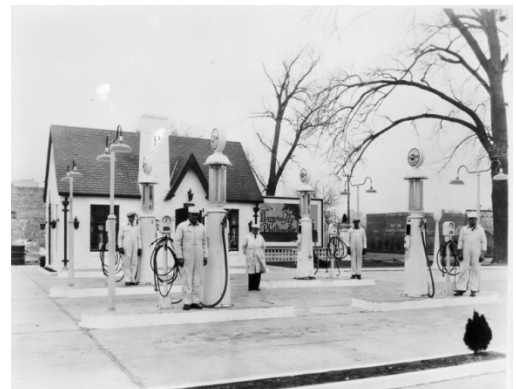
1 st Phillips 66 Filling Station November 19, 1927 - Wichita, Kansas
