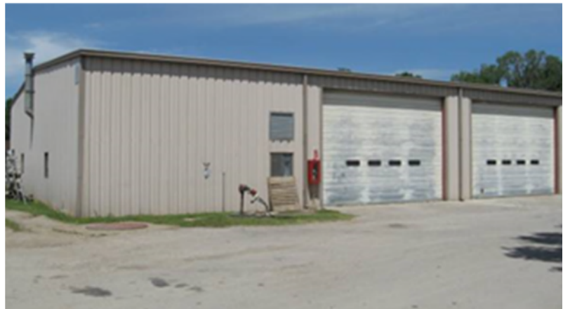
Figure TM2.2-34 Maintenance Building
