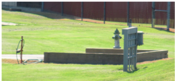
Figure TM2.2-10 Septage Receiving Station
