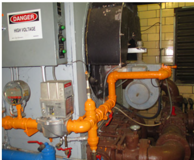
Figure TM2.2-28 Digester Heaters
