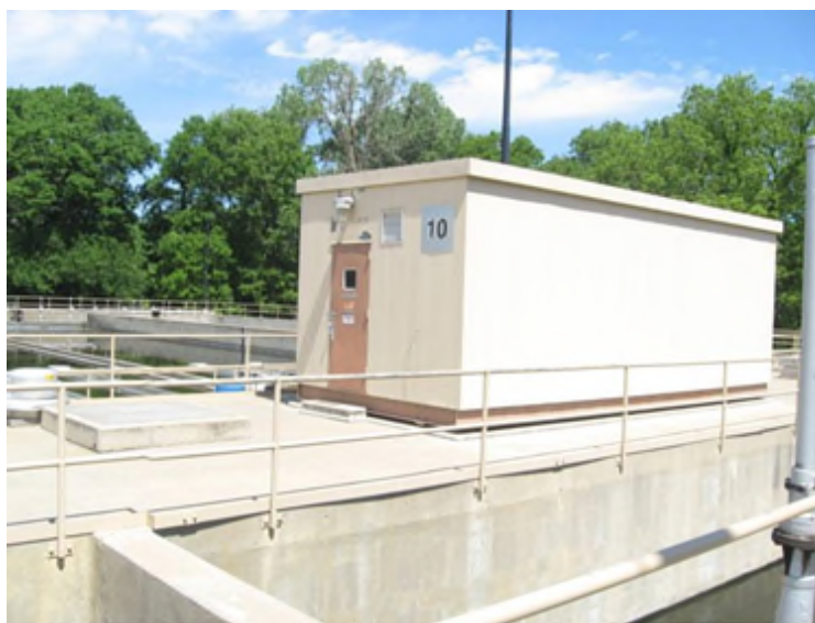
Figure TM2.2-19 Return Sludge Pump Station
