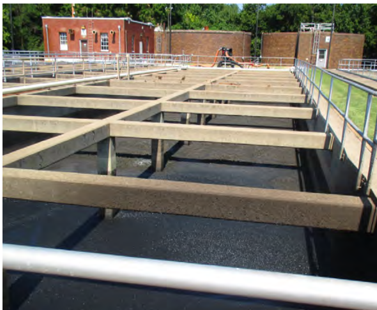
Figure TM2.2-30 Sludge Storage Basin
