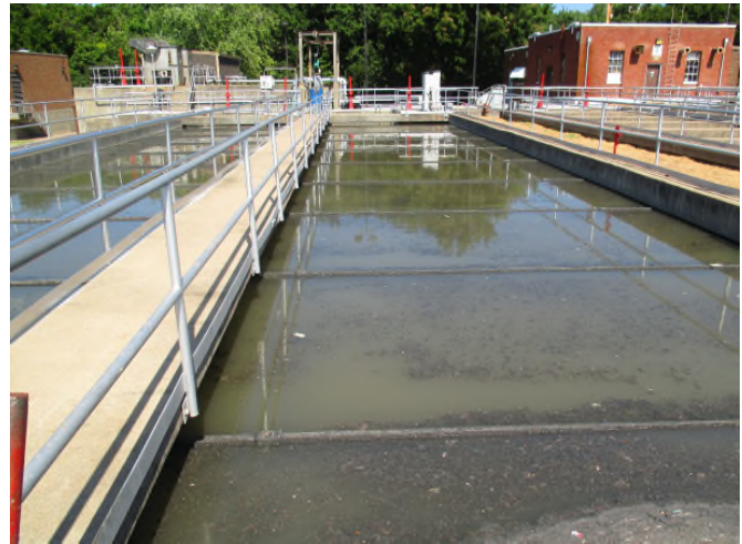
Figure TM2.2-11 Primary Clarifiers
