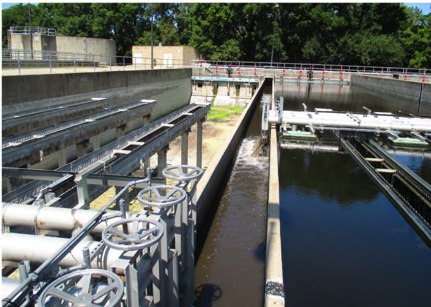
Figure TM2.2-16 Rectangular Clarifiers
