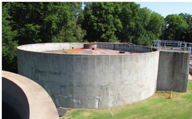
Figure TM2.2-27 Secondary Digester (AD#3)
