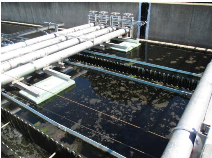
Figure TM2.2-18 Final Clarifier #2
