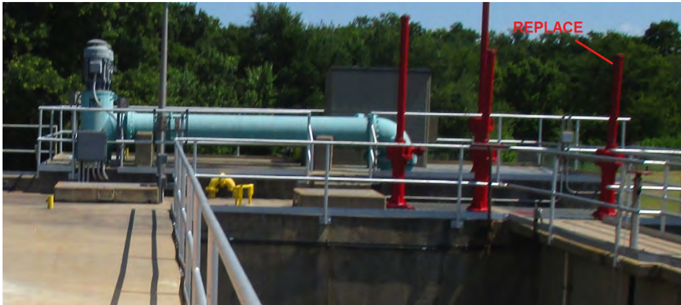
Figure TM2.2-21 Effluent Pump Station- 1 of 3 Gates to be Replaced
