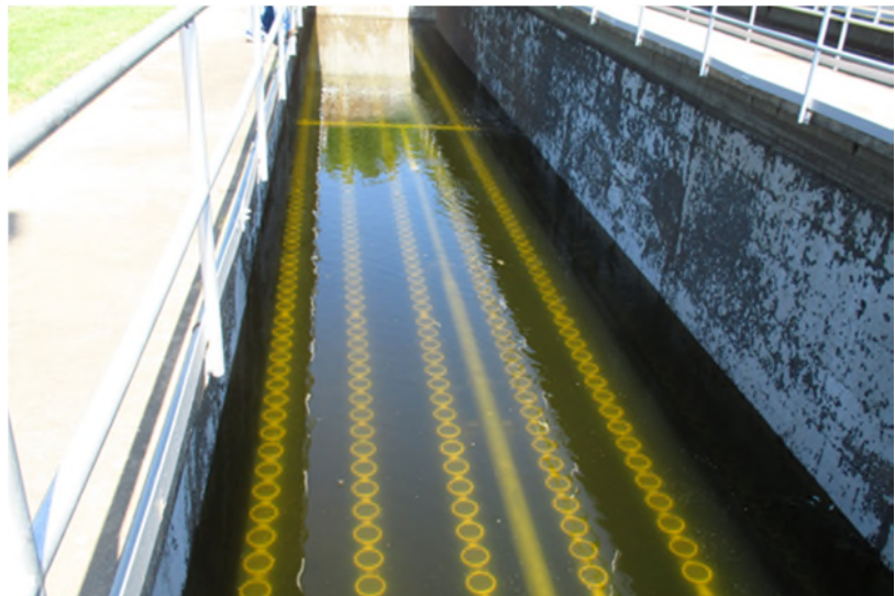
Figure TM2.2-15 Aeration Basin- Ceramic Disc Diffusers
