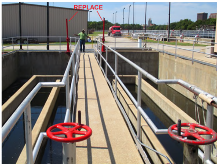
Figure TM2.2-22 Chlorine Contact Basins 2 of 3 to be Replaced
