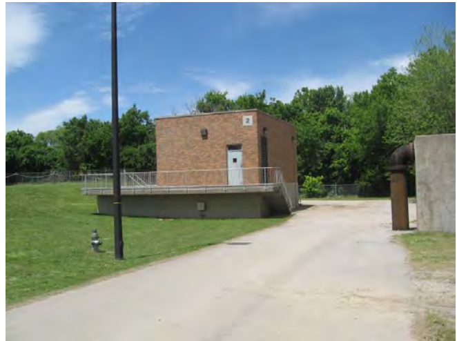
Figure TM2.2-1 Chickasaw Lift Station
