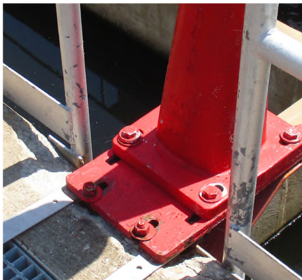
Figure TM2.2-23 Concrete Failure by Stand
