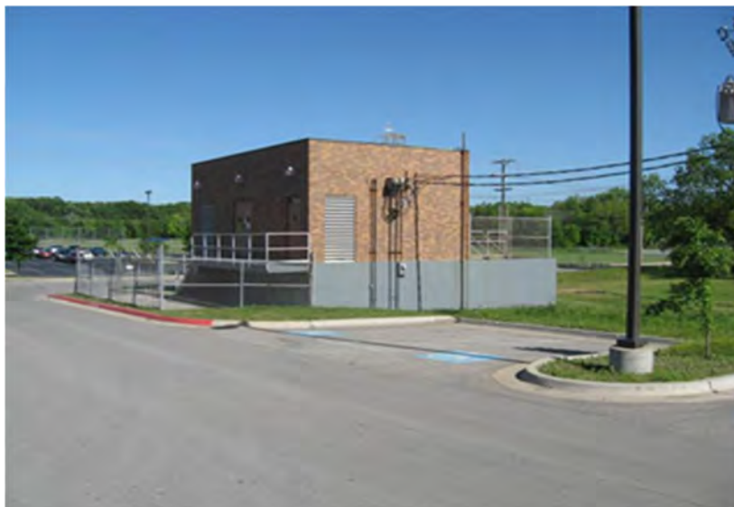
Figure TM3.5 - Shawnee Lift Station
