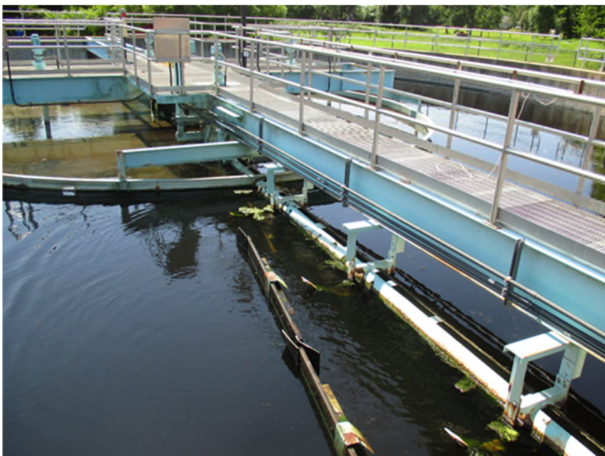
Figure TM2.2-17 Final Clarifier #4
