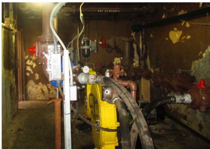
Figure TM2.2-13 Peristaltic Pumps
