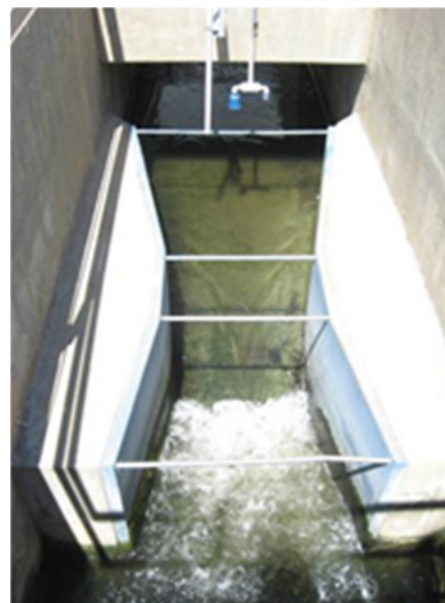
Figure TM2.2-20 Parshall Flume
