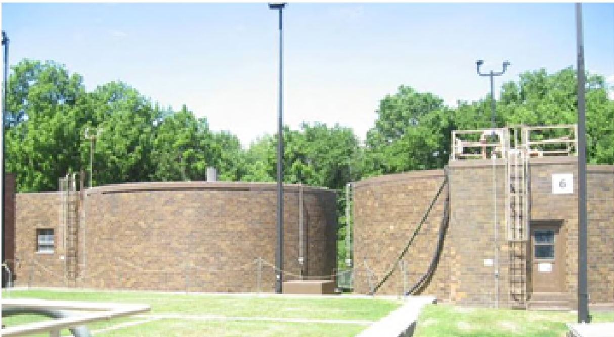
Figure TM2.2-25 Primary Digesters
