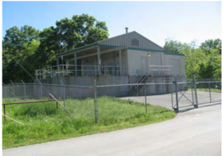
Figure TM3.4 - Limestone Lift Station
