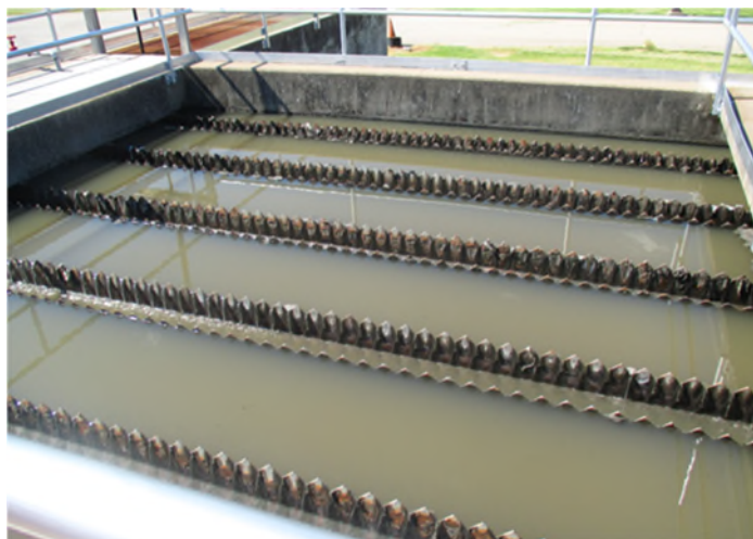
Figure TM2.2-12 Effluent Channels and Weirs
