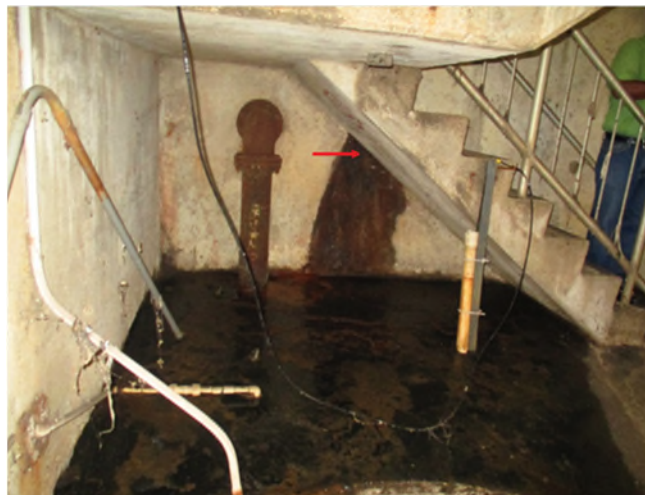
Figure TM2.2-3 Groundwater Seepage through Walls
