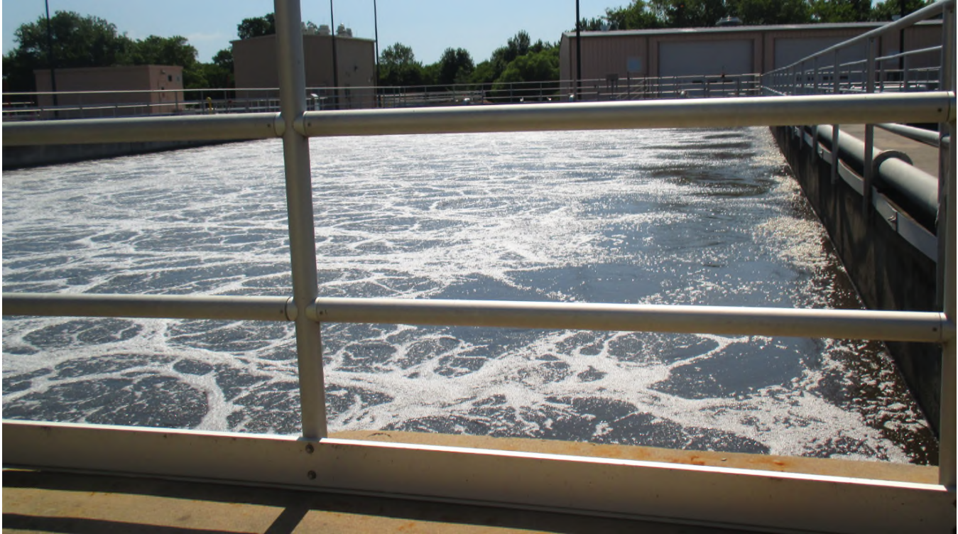
Figure TM2.2-14 Aeration Basin
