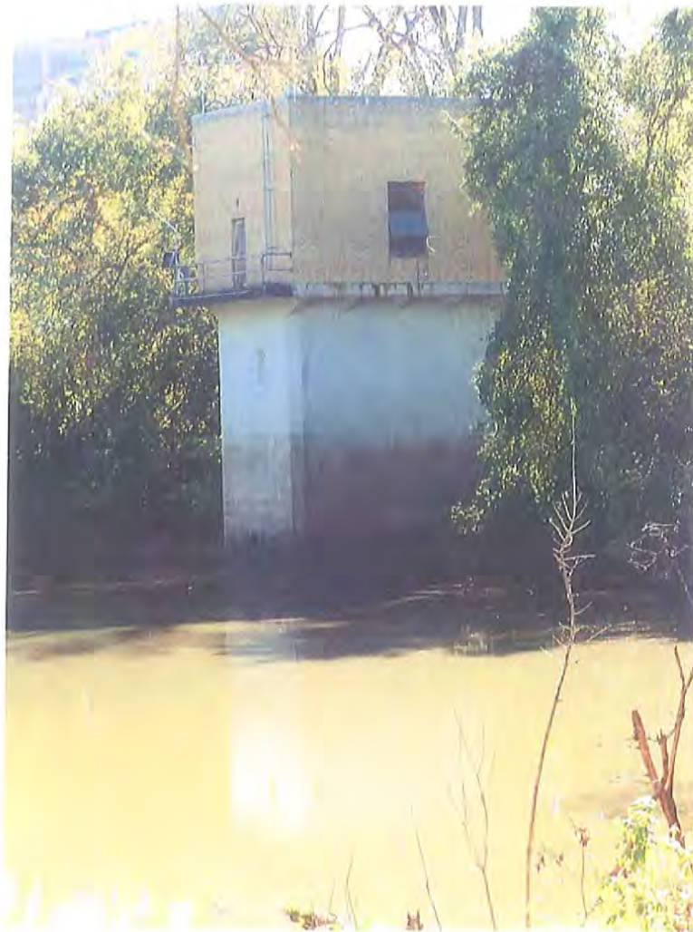
Photograph 8: City of Bartlesville, Caney River Intake Structure
