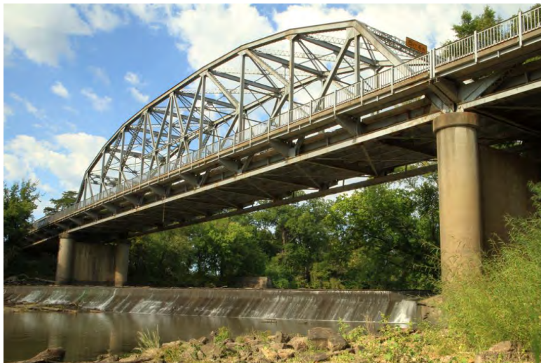
Pictured: low-head dam on the Caney River underneath Oklahoma State Highway 123 (ODOT, 2016)
