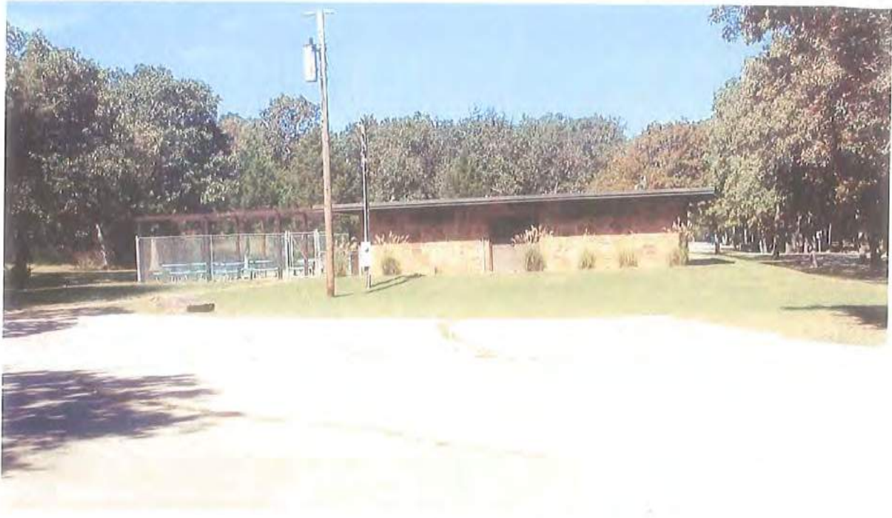
Photograph 5: Osage Hills State Park Swimming Pool
