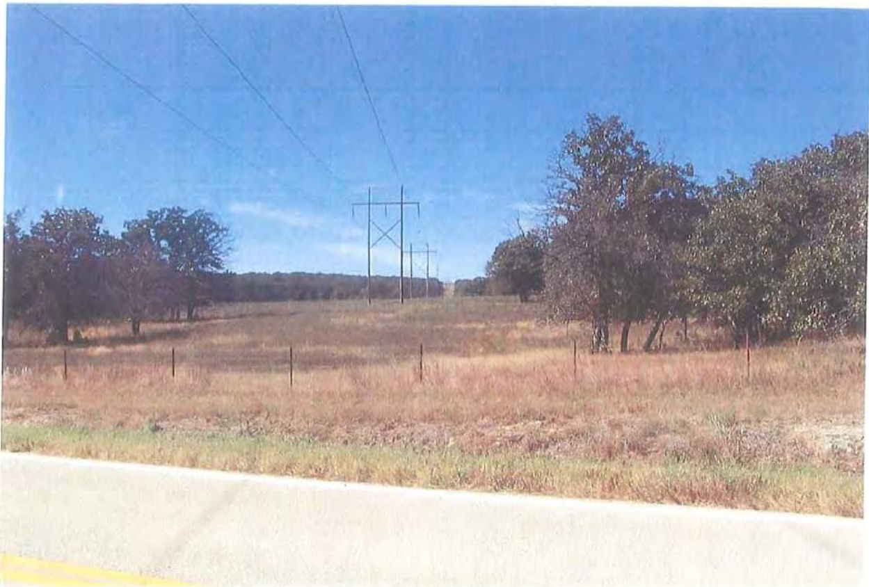
Photograph 3: Highway 99 Power Transmission Line Crossing
