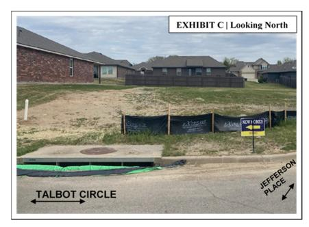
However, a large storm sewer inlet on Talbot Circle, shown in **Exhibit C**, leaves no room for a driveway. Therefore, Tanner Consulting, on behalf of D.R. Horton, is requesting approval to modify the Limits of No Access that are shown on the recorded plat to allow the driveway to be located on Jefferson Place. Their proposed plat amendment document and plot plan are attached as **Exhibit E**.
