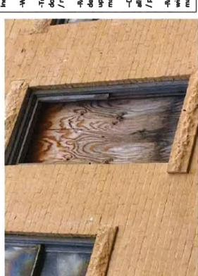
Corrective Action(s): Including: -Weatherproof as required;
