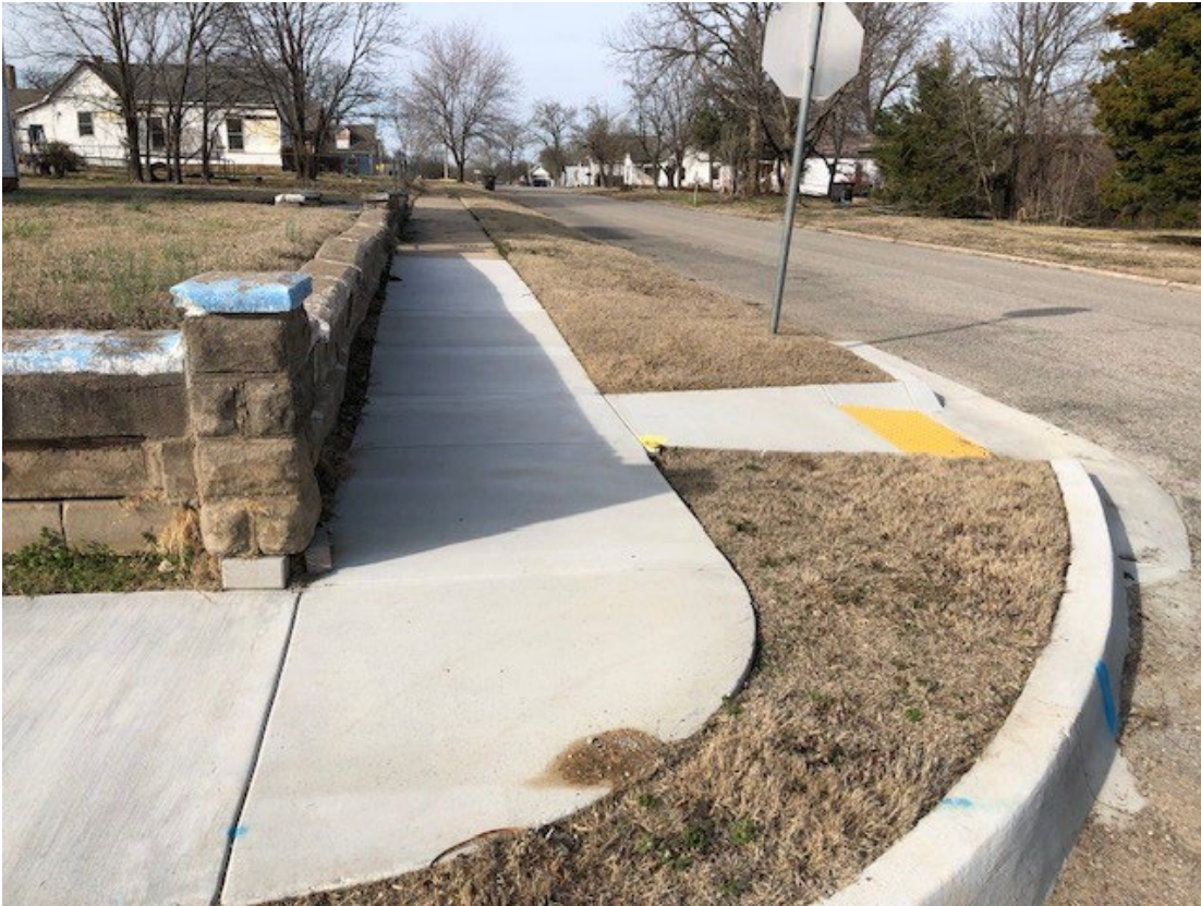
Cheyenne Ave (Looking North)
