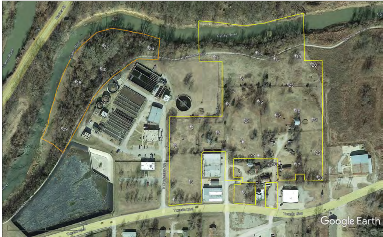
The two APE portions near the existing WWTP and STPs dug within these areas.
