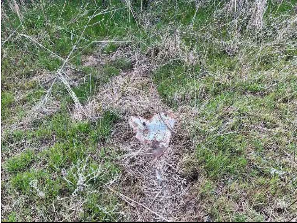
Metal road culvert
