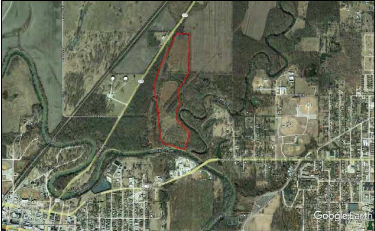
2015 aerial photograph of the site boundaries
