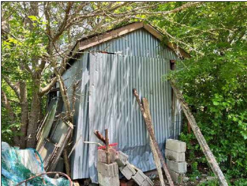
Standing structure used for storage, documented on an HPRIF
