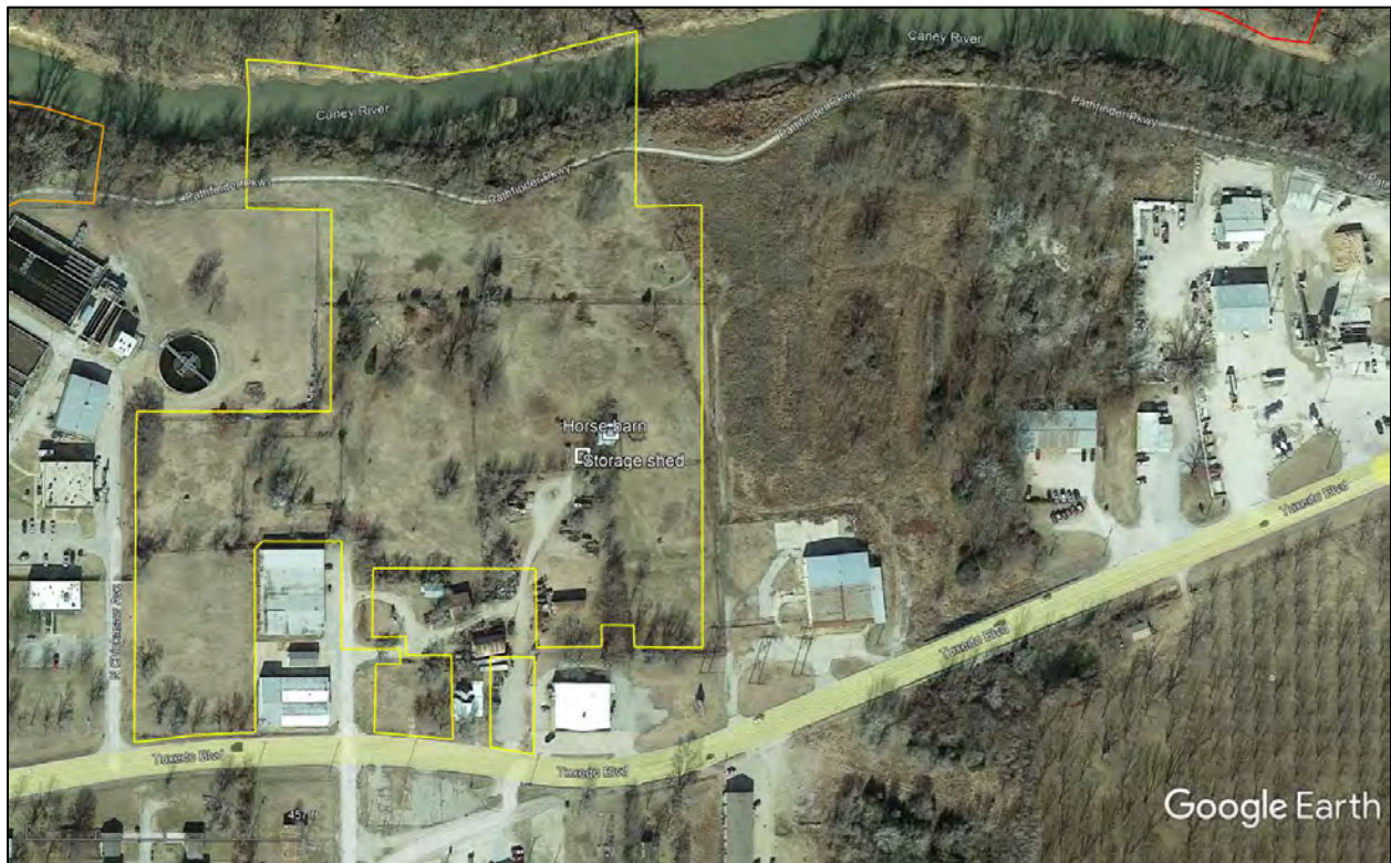
Aerial photograph of the location of the two structures in Bartlesville, OK
