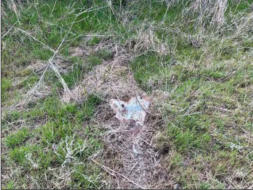
Metal road culvert
