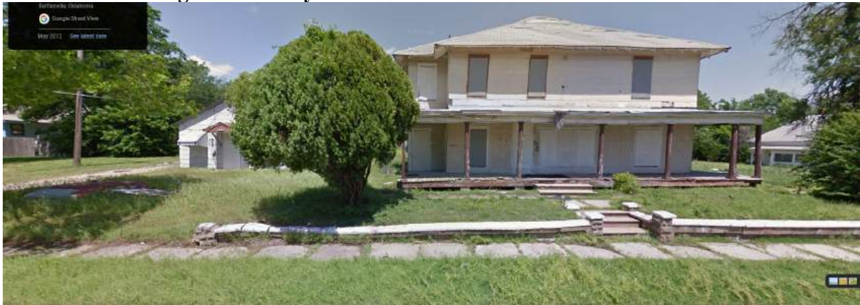
5 th Street—Looking North—May 2012
