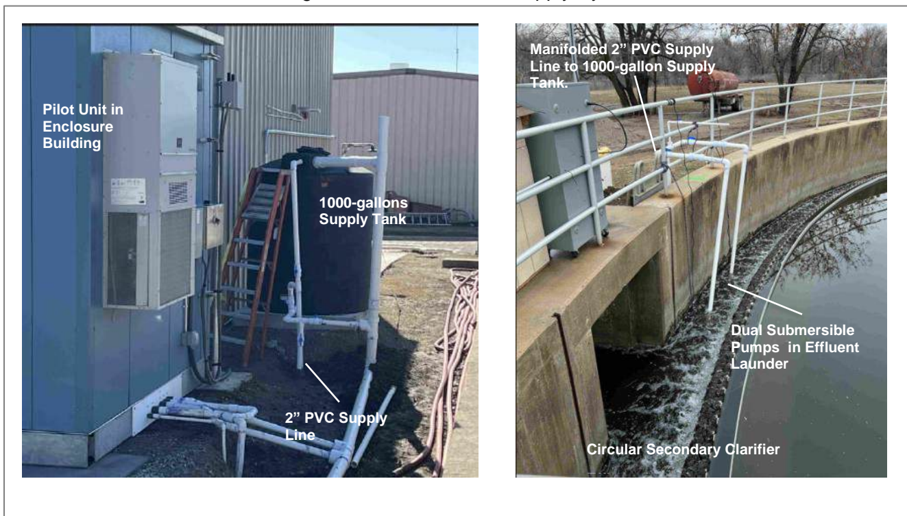
Figure 2-4 Source Water Supply System
