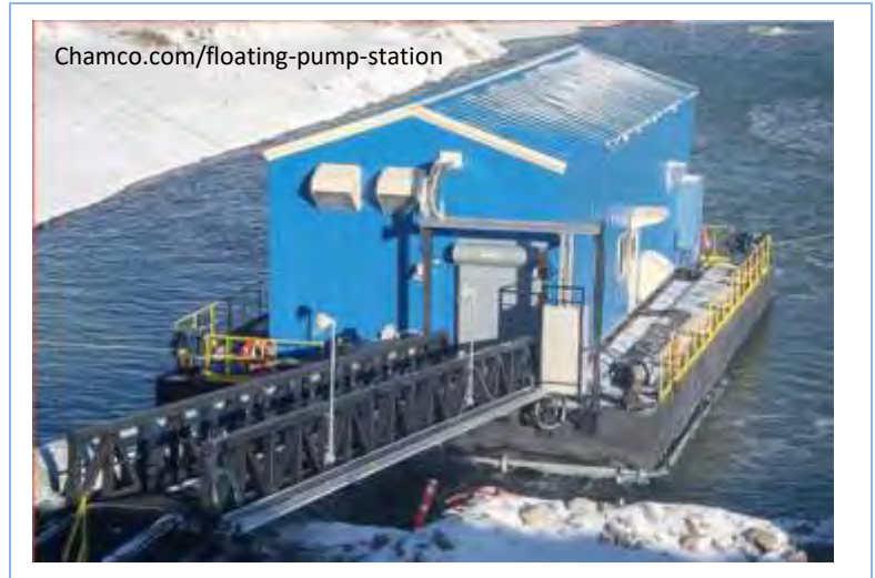
Figure 2-12 Floating Intake Combined with Pump Station
