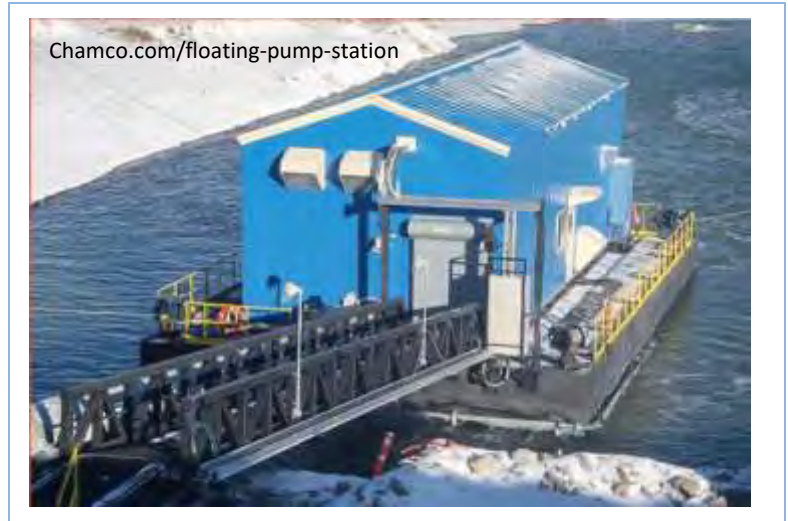
Figure 2-12 Floating Intake Combined with Pump Station
